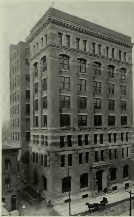
TELEPHONE BUILDING, MILWAUKEE. Faced with wire cut dark red brick, made by Western Brick Company. A. C. Eschweiler, Architect.
